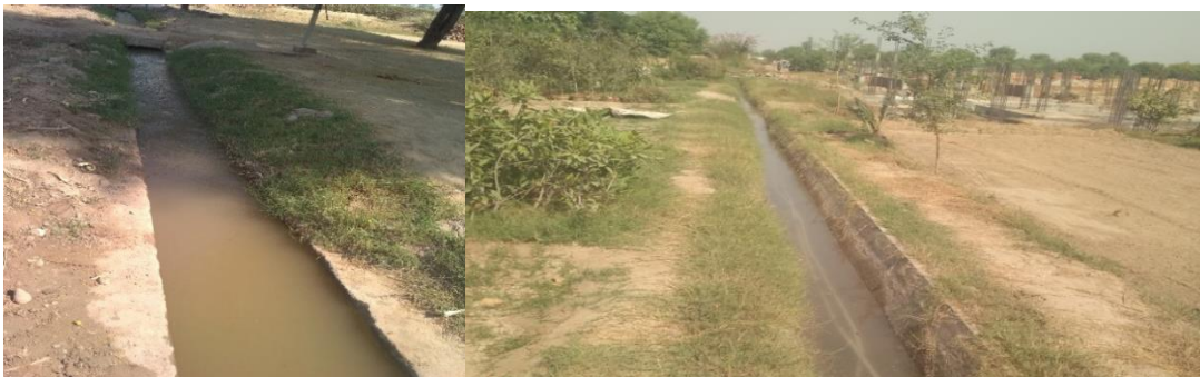
Figure 18: Cemented Water Channels
