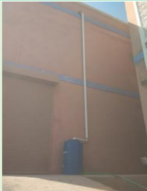
Automatic on/off taps as a policy to replace manual taps (left), Rainwater Harvesting System (Right)
